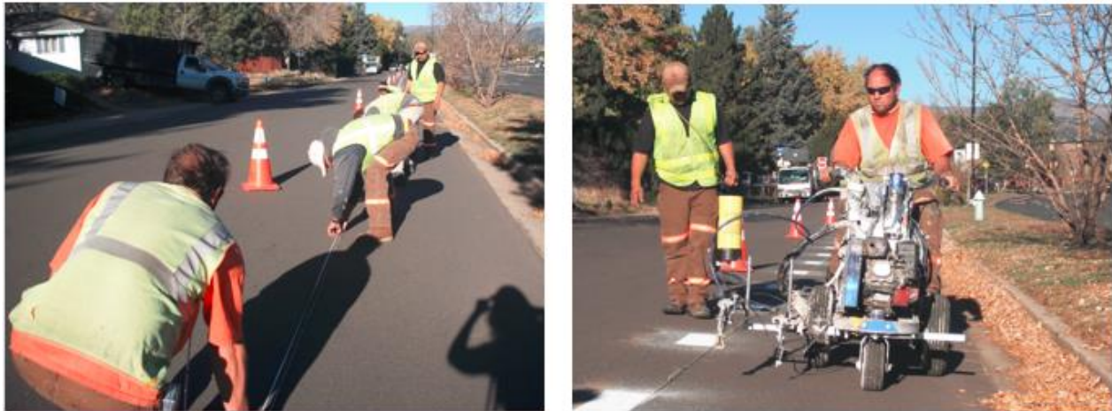
Figure 3: Harvard DBL installation (October 2014)
