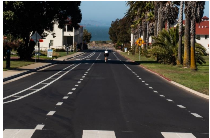
Figure 1b: Graham Street After ABL Installation (Looking North)
