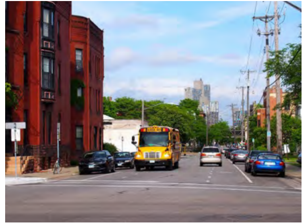
Figure 7-10: Two oncoming vehicles negotiating on 14 th Street East between Park Avenue South and Chicago Avenue South within a 14-foot two-way travel lane after installation
