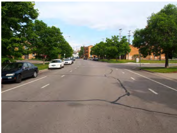
Figure 7-5: Grant Street East facing east at Portland Avenue South after installation with a 20-foot two-way travel lane
