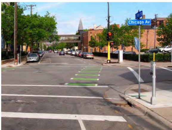
Figure 7-19: Green bicycle lane conflict markings installed on 14 th Street East at Chicago Avenue South
