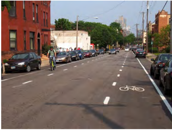
Figure 7-9: A westbound bicyclist riding on 14 th Street East between Park Avenue South and Chicago Avenue South adjacent to a 14-foot two-way travel lane after installation
