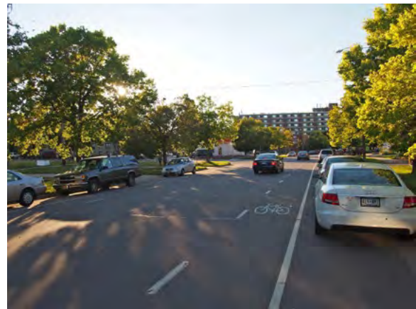
Figure 7-6: Grant Street East facing west at Park Avenue South after installation with a 20-foot two-way travel lane
